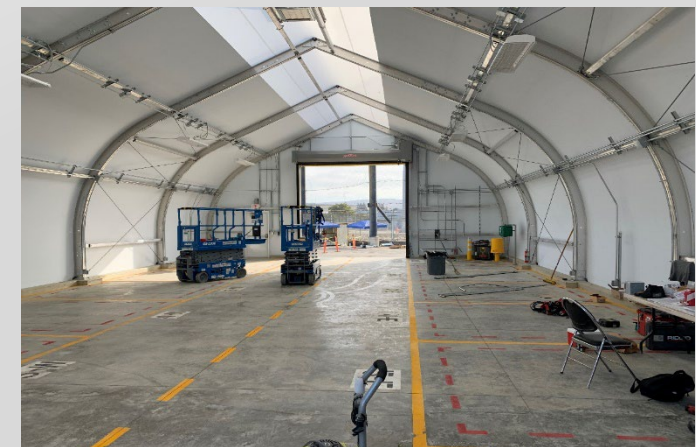
New Superblock Storage Area Installation, LLNL
