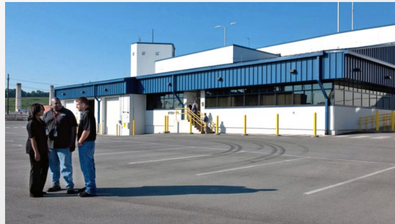
Highly Enriched Uranium Materials Facility, Y-12
