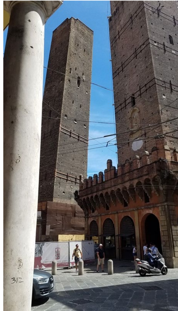
Figure 3: The Bologna Leaning Towers 7
