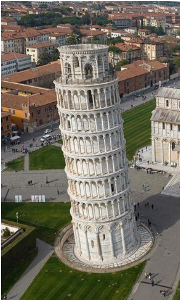
Figure 2: The Leaning Tower of Pisa went sideways because its builders didn't understand that the ground below one side was softer than the other 6
