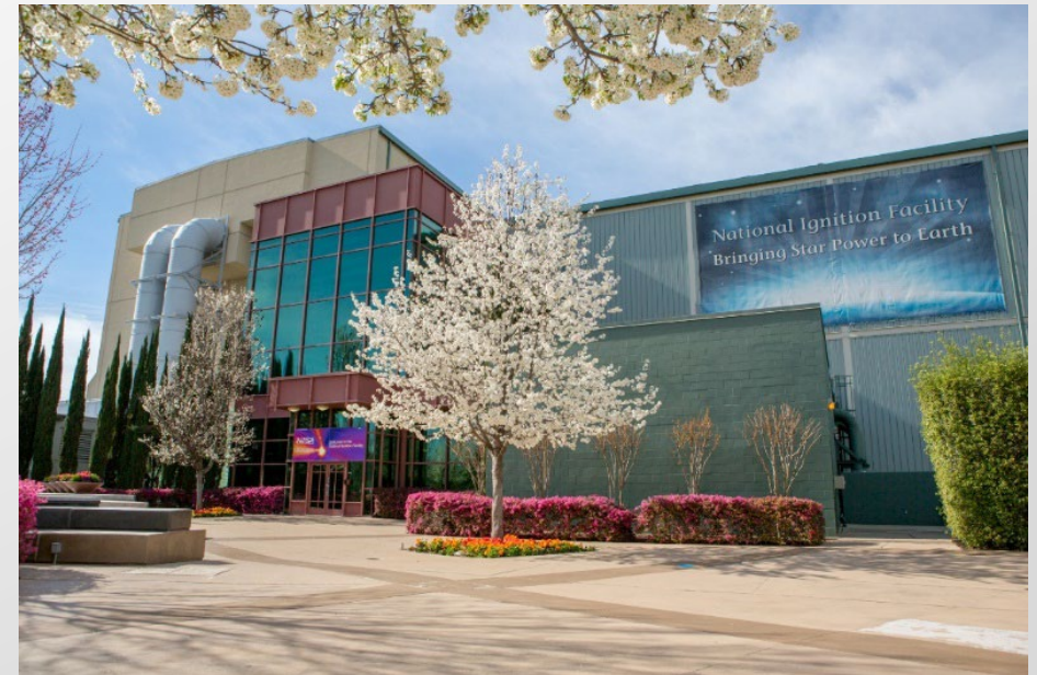
NNSA Capital Projects range from office buildings to the National Ignition Facility (Pictured Above)
