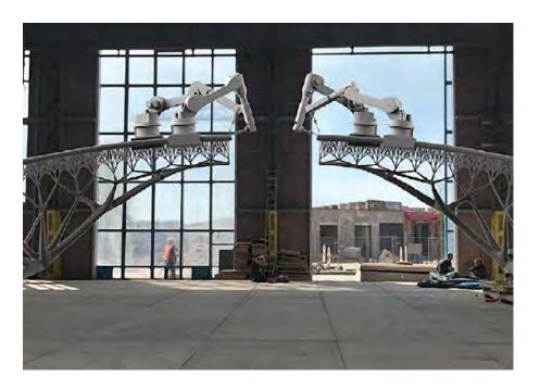
A Dutch startup is using 3D printing to produce a large, complex structure to build a bridge made of printed steel
