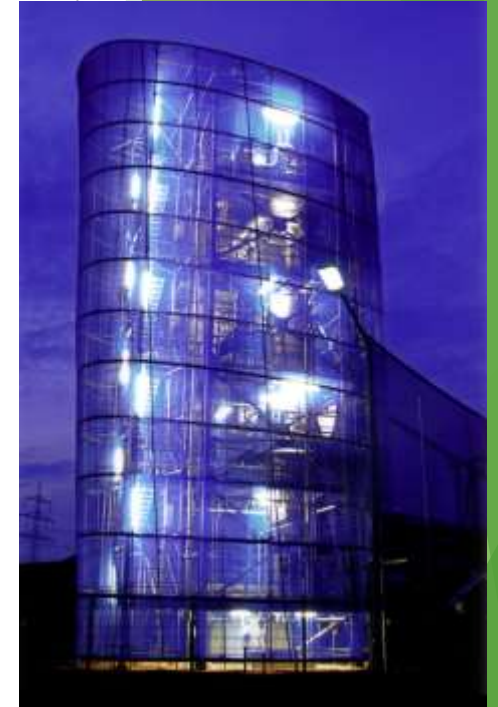
Current Concord Blue waste-to-power facility in Herten, Germany
