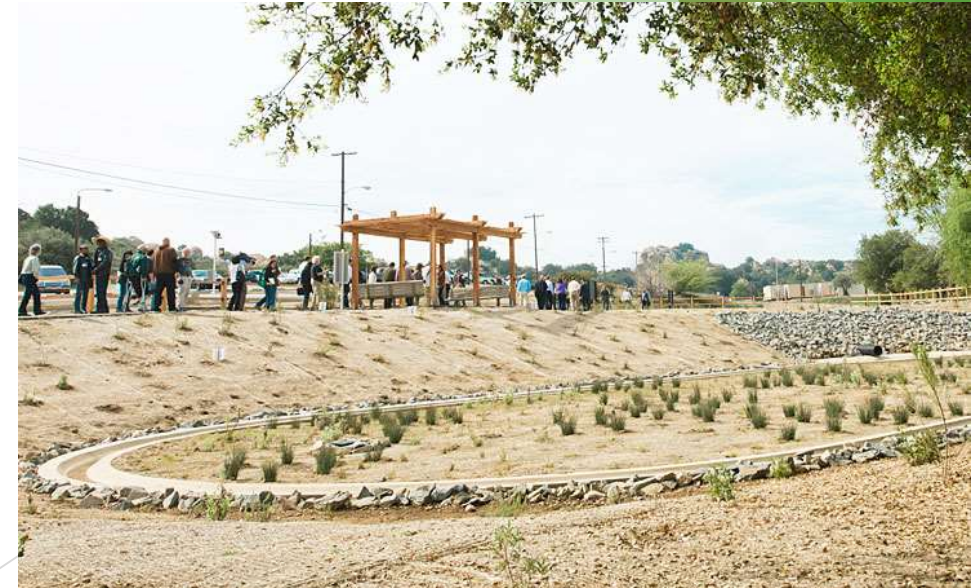
A biofilter storm water treatment system at Boeing Santa Susana site
